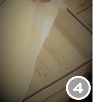
Begin in a corner. Insert about 2 inches of the fabric panel into the channel.
